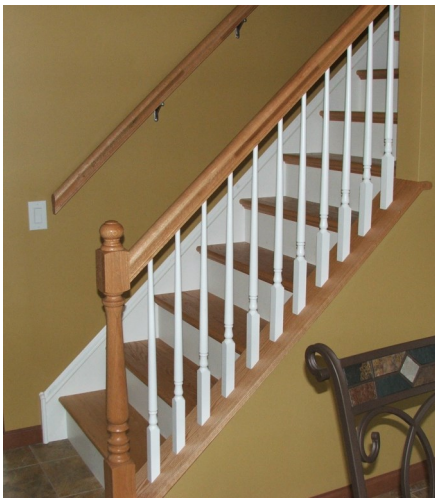
Stained oak treads with white risers/skirtboard
